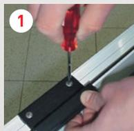
Installation of the chain coupling to the mobile wing
